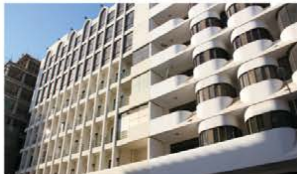
Trading Building Air Cooled Screw Chiller Oman
